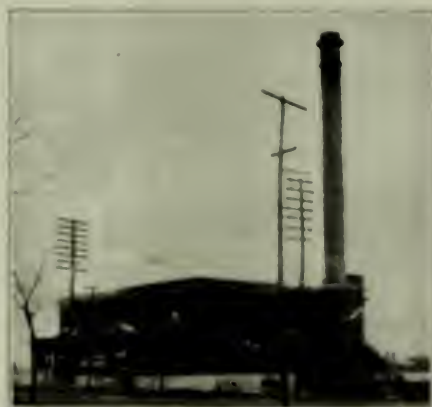
FIG. 2. POWER HOUSE OF THE ST. CLAIR TUNNEL COMPANY
